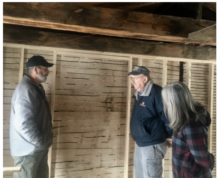
Gardner Norcross and board members Ron Remick Sr. and Jennifer Kelley Reed admire some of the old wide-board split lath we found. We will keep sections of it visible.
